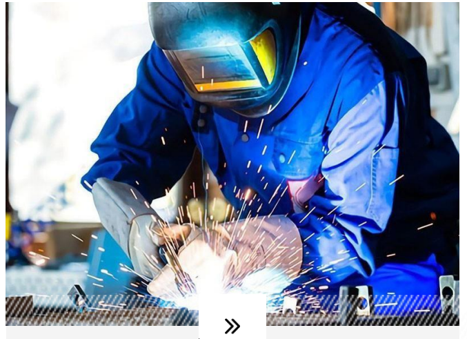
Steel Welding / Fabrication Works
